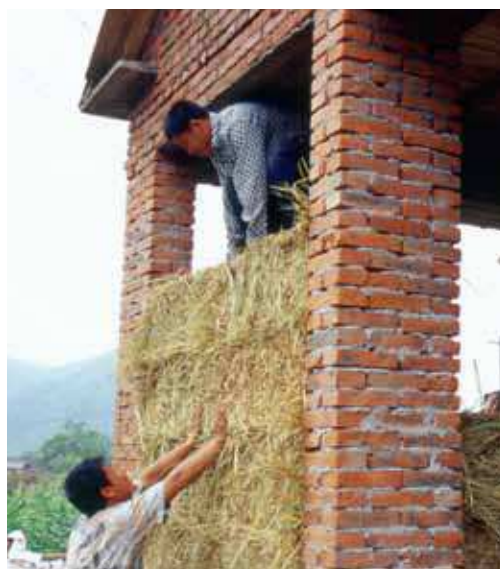
Stacking straw bales between brick columns, Heilongjiang, China. © Kelly Lerner, One World Design Architecture.
