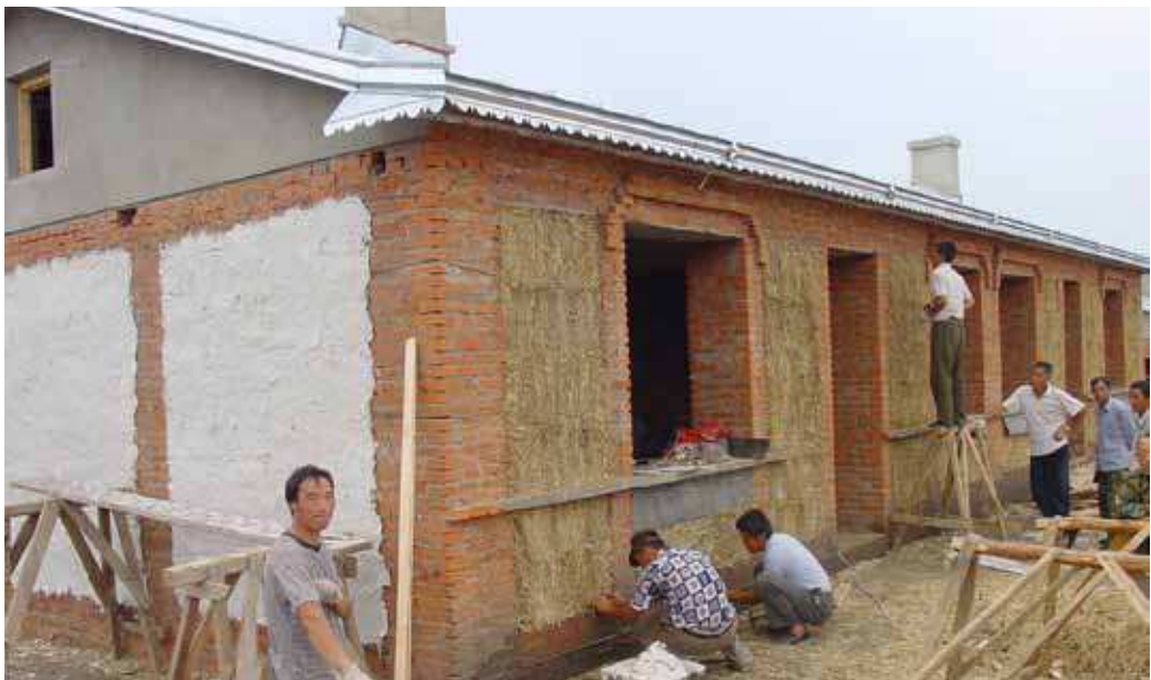
Strawbale house with brick frame under construction. © Kelly Lerner, One World Design Architecture.
