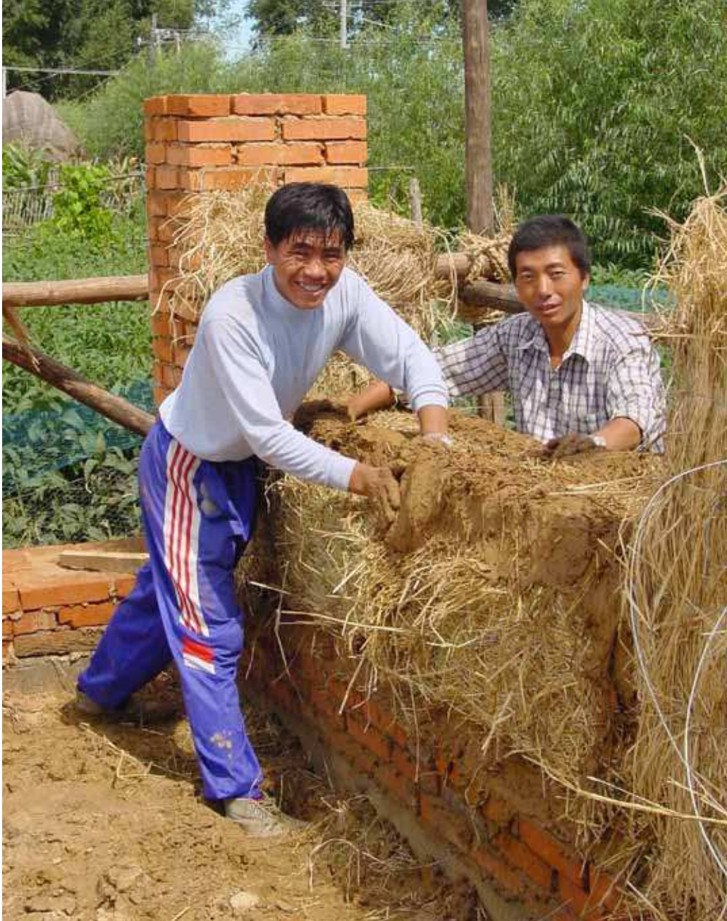
Stacking strawbale walls with earthen mortar, Jilin, China. © Kelly Lerner, One World Design Architecture.
