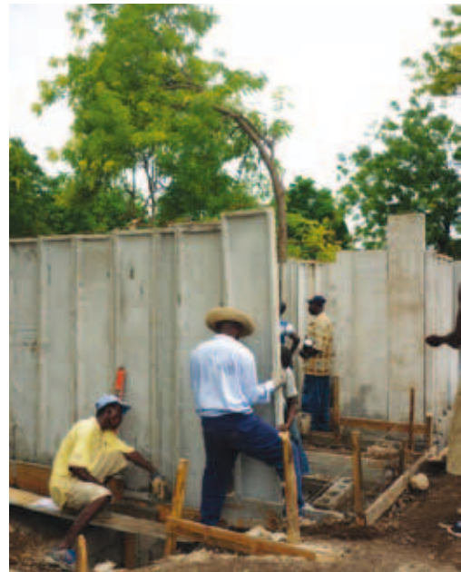
One mason and three helpers assemble the house. © Ecosur.
